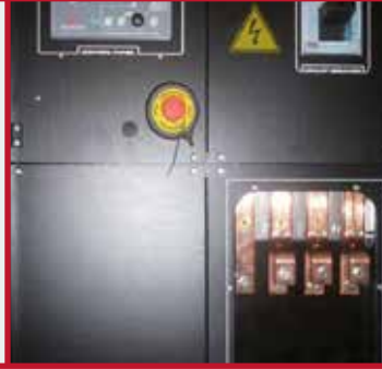
POWER TERMINALS (STANDARD FROM MSW275V)
